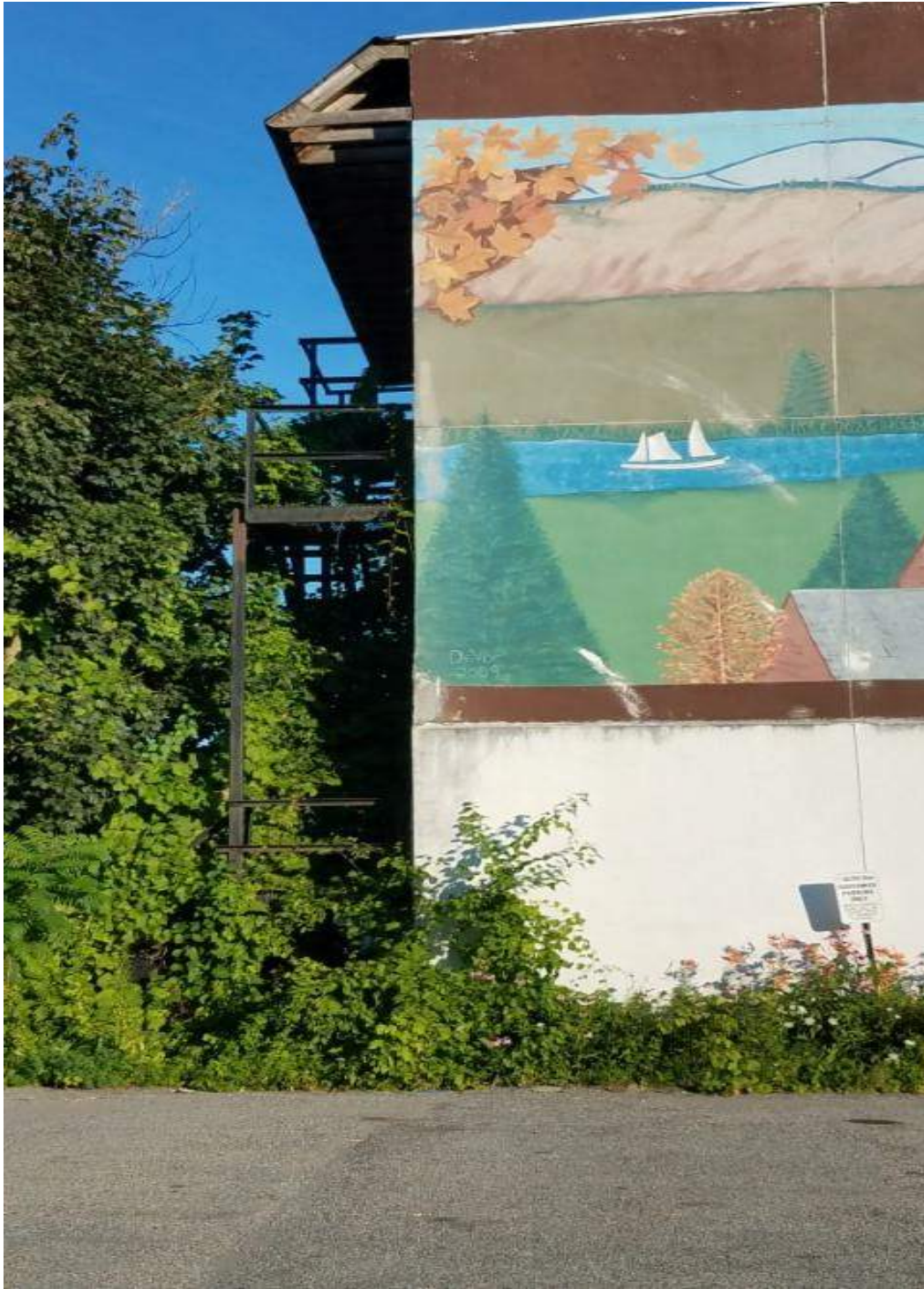
140 Broadway and its faded mural facing southbound traffic through Fort Edward's Downtown at the strategic Route 4 and East Street intersection. Note the condition of the fire escape and the temporary roof bracing installed several years ago to prevent interior water damage and brick failure in an attempt to save the building for a developer.
